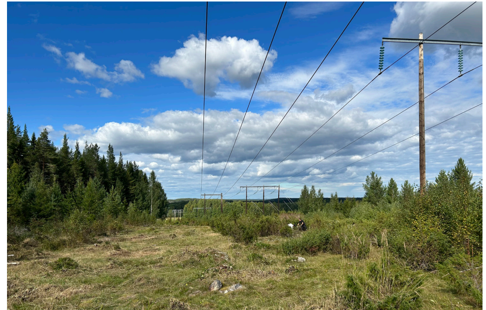
Maintenance of the core areas in the power line corridor
