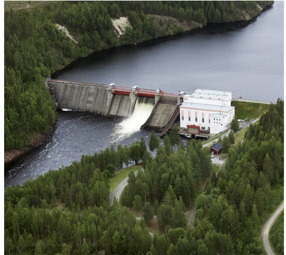
Hydroelectric power generation is part of the EU Taxonomy
